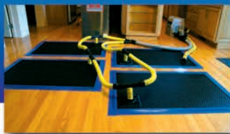
Hardwood Floor Drying
