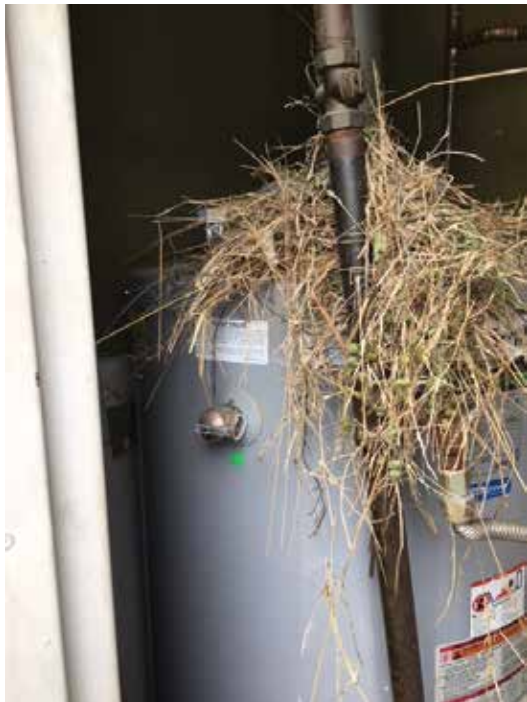
The remainder of the straw that was packed around this heater for insulation.
