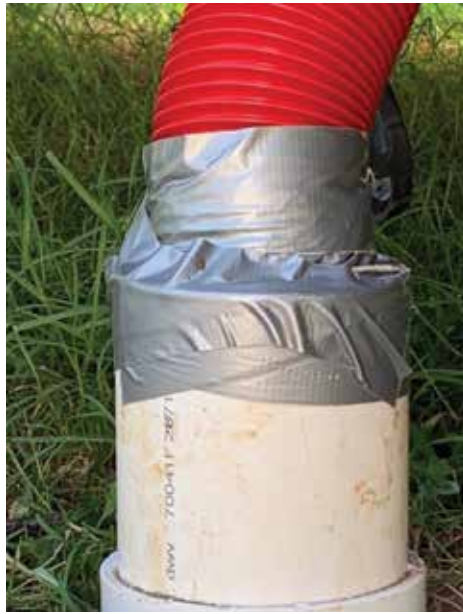
When you use unapproved materials for drainage it is easier to connect them with duct tape.
