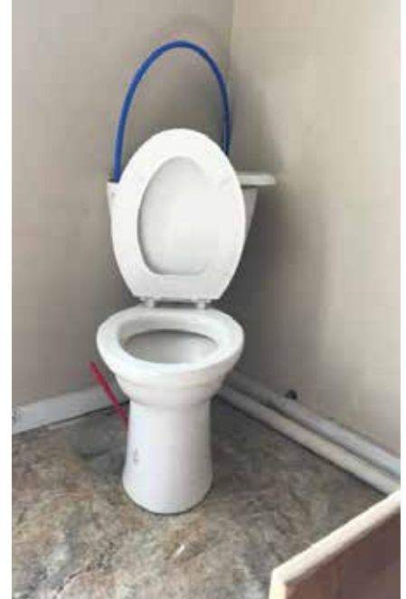
Why run the PEX to the ballcock when you can just stick it in the tank?
